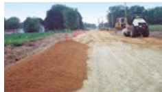
38th St - During Reconstruction
